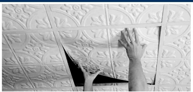
• Determine the number of tiles required. When installing in an existing suspended ceiling grid, count the number of whole panels and border panels needed. If installing a new grid system, perform the same count from your grid layout plan.
